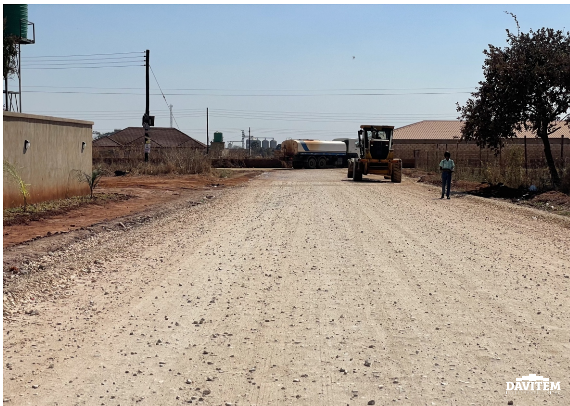
Stock Piling of Gravel
