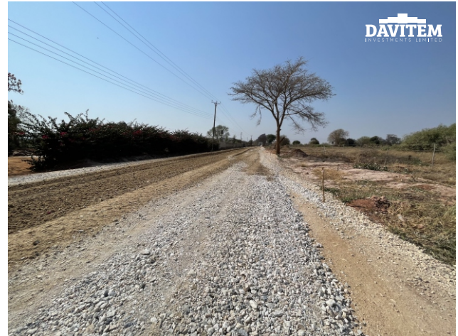
Processing of Gravel
